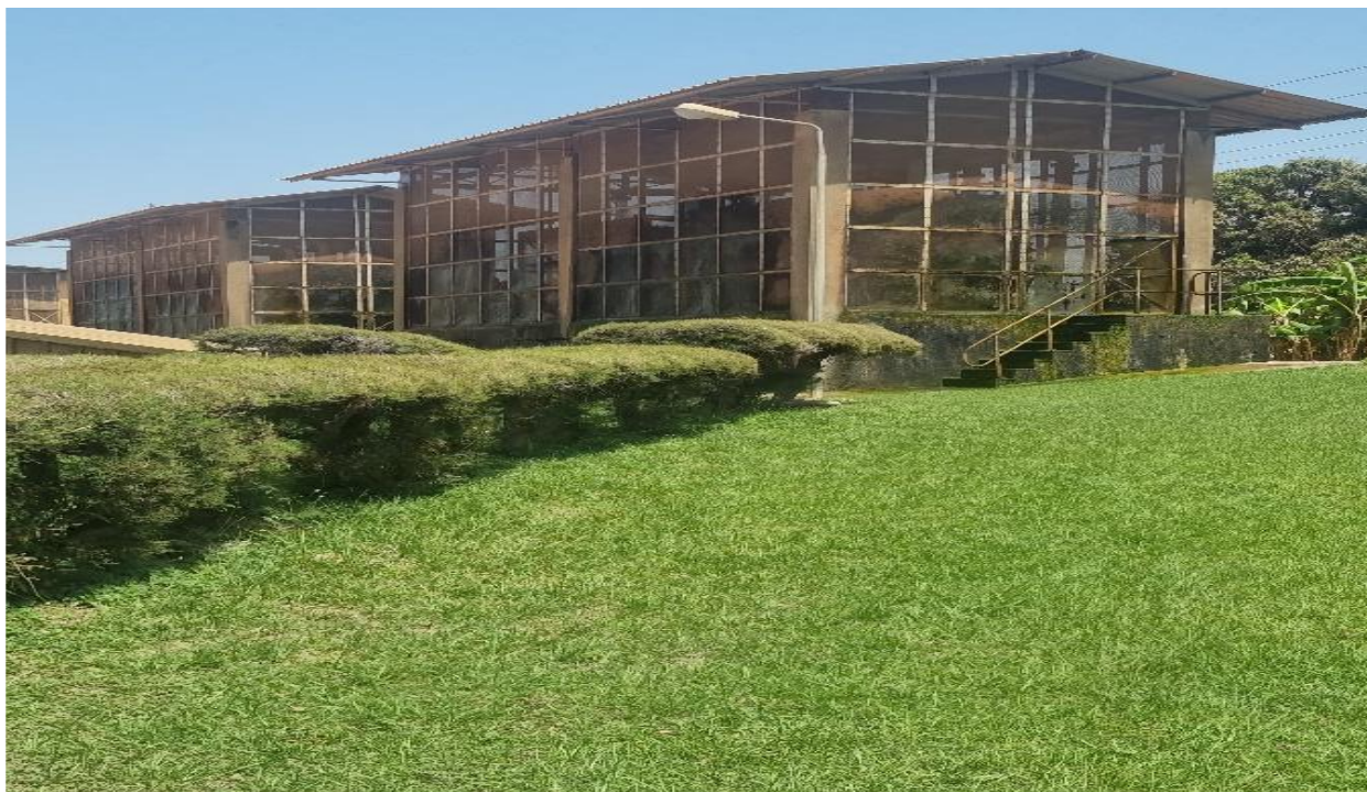
Figure 2.1: An aeration facility at one of NAWEC's treatment plants
